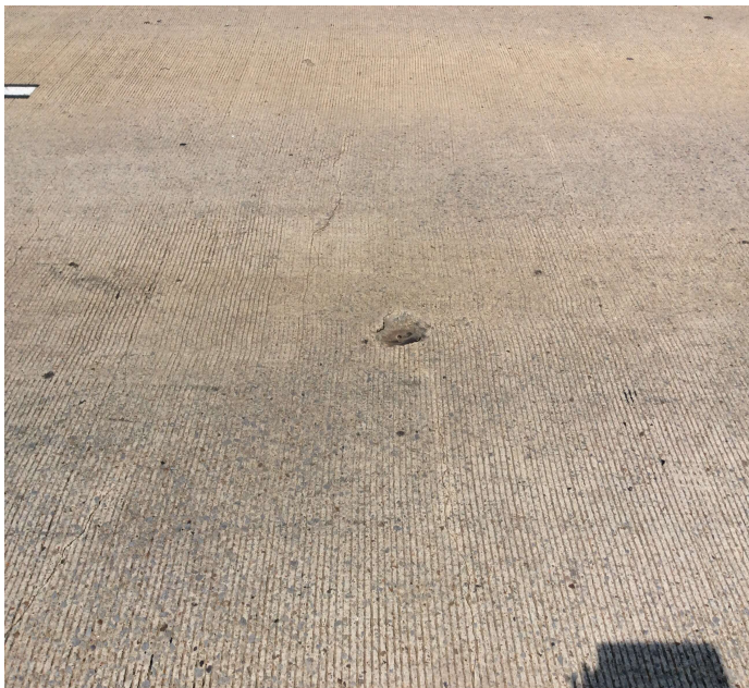
PHOTO 1 Description Span 4 debris cast in the deck.
